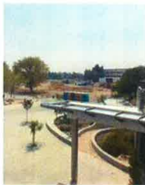
Photo 4 - Construction view from second floor H&S building
