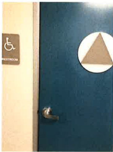
Photo 21 – Unisex Restroom: Consider Using an Occupied Sign.
