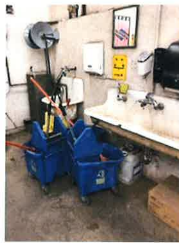
Photo 10 – Obstructed Eye Station
