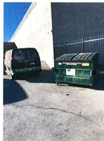
Photo 22 – Obstructed Emergency Exit
