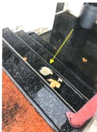
Photo 8 – Visitor Dugout Stairs
