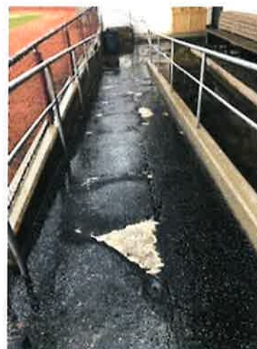
Photo 6 – Home Dugout Ramp
